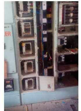
Retrofitting of ACB/MCCB/SFU
