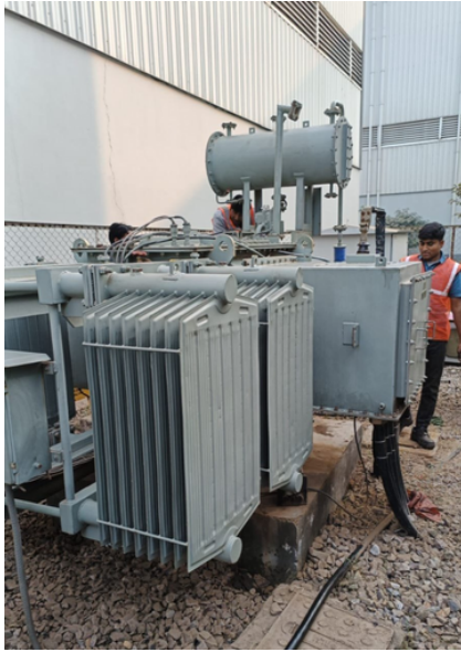
Dehydration and filtration of Transformer
