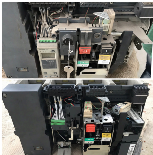
Servicing and Overhauling of ACB
