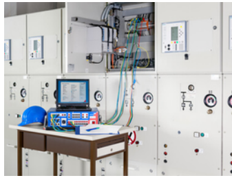
Testing of Protection Relay
