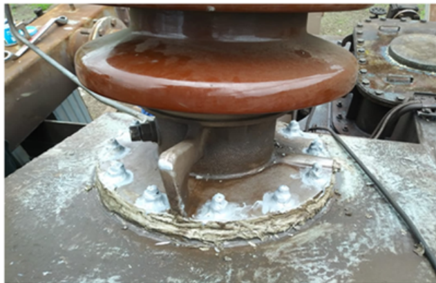
Transformer Oil Leakage Arresting
