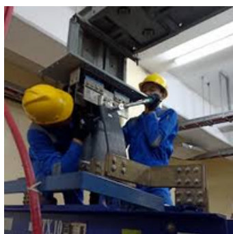
Maintenance of Bus duct
