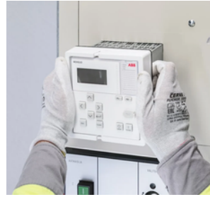
Retrofitting work of protection Relay
